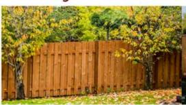
With a Good Neighbor fence, cedar boards are installed on alternating sides of the rails, giving the fence the same appearance from both sides.
