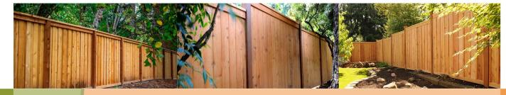
Our Picture Frame Fence: Cedar boards mounted side by side with a minimal gap to allow for expansion and contraction. Overlapped boards are optional. Fence boards are installed between the posts. Rails are place at the top and bottom of the fence and Horizontal 1x4's or 1x6's are placed at the top and bottom to finish the look. A 2x6 or 2x4 continuous cap is placed on top.
