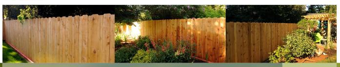
Our Picture Frame Fence: Cedar boards mounted side by side with a minimal gap to allow for expansion and contraction. Overlapped boards are optional. Fence boards are installed between the posts. Rails are place at the top and bottom of the fence and Horizontal 1x4's or 1x6's are placed at the top and bottom to finish the look. A 2x6 or 2x4 continuous cap is placed on top.
